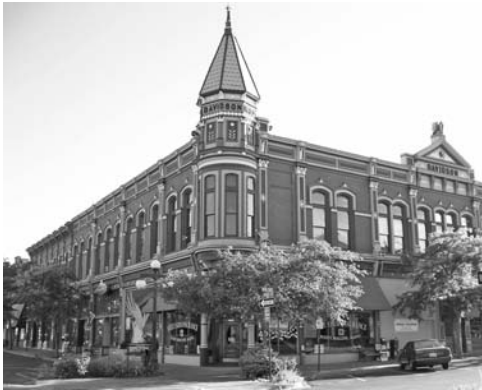
The Italianate-style Davidson Building, built in 1889. (Photo courtesy of CTED)
