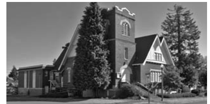
Trinity United Methodist Church, 1913–1915 (rehabilitation in process)
