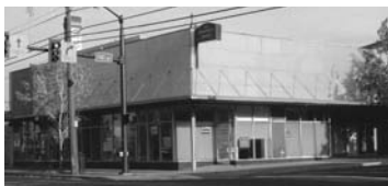
The 1920s Pantorium Building underwent misguided modernization over the years.
