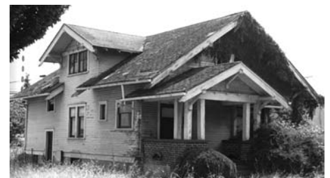
This 1916 Tacoma bungalow is being salvaged to demonstrate green preservation practices.
