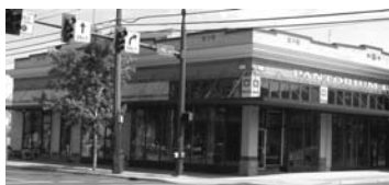
In 2005, the Pantorium was restored, exposing the original parapet exterior and transom windows.
