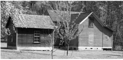
The Olson House and weaving shed are part of Auburn's Mary Olson Farm, a 60-acre farmstead that will serve as an interpretive site. (Courtesy of BOLA Architecture + Planning)
